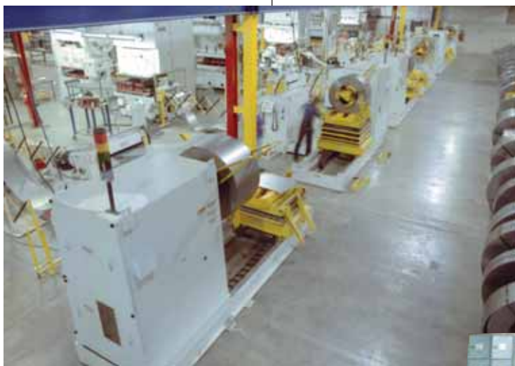
Coil reels with integrated coil cars head up each of seven new press lines.
